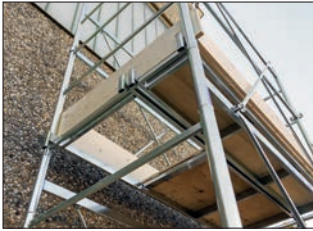
Two-part work platform (840x1670 mm) with trapdoor and toe boards to prevent falling objects.
