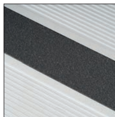
Wide steps with slip-proof insert depth: 210 mm.
